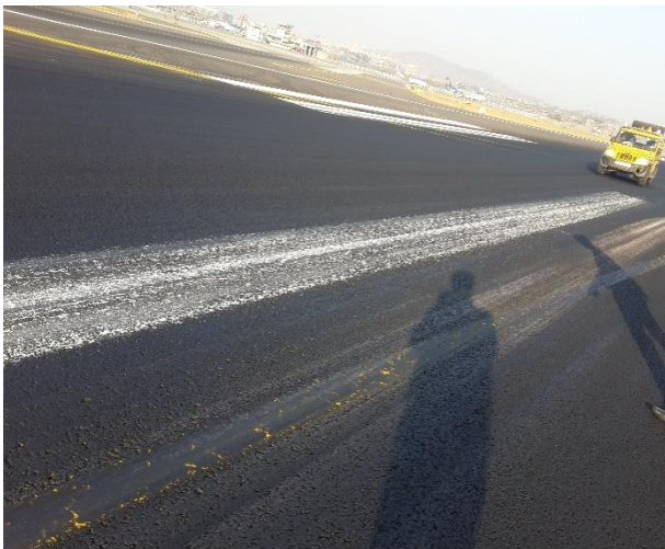
Belly scrape marks on the runway
