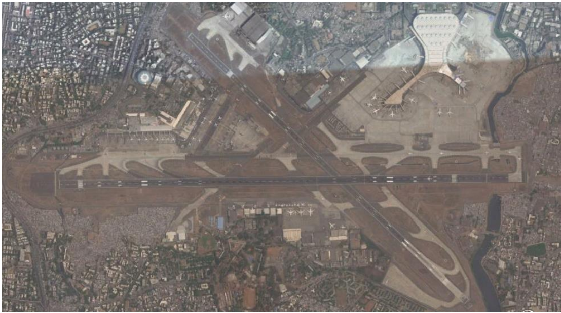
Figure: Chhatrapati Shivaji International Airport, Mumbai
